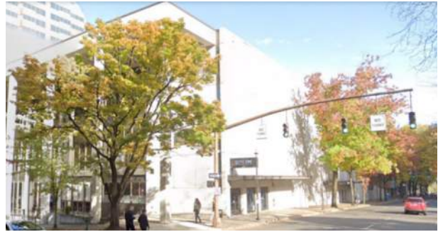
Façade along Southwest Market Street at Southwest Third Avenue
